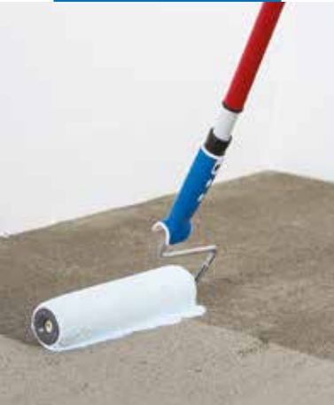
Primer application on the substrate
