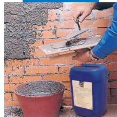
Spatter - dash coat modified with Planicrete SP
