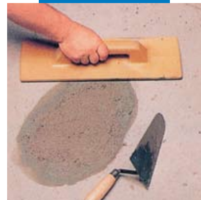
Floor patching: final smoothing
