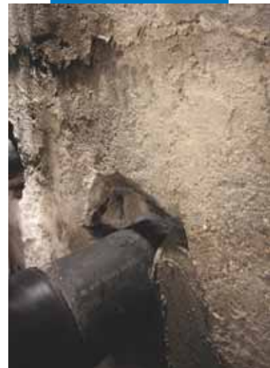
Confining Mapeproof Swell with Mapegrout T40
