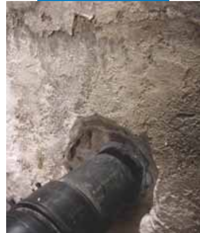
Mapeproof Swell after application
