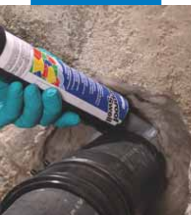
Applying Mapeproof Swell around a pipe
