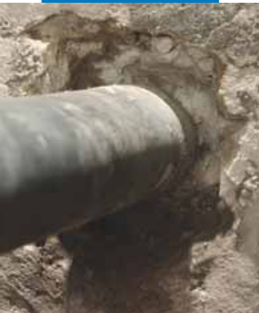
Demolition of the structure around a pipe
