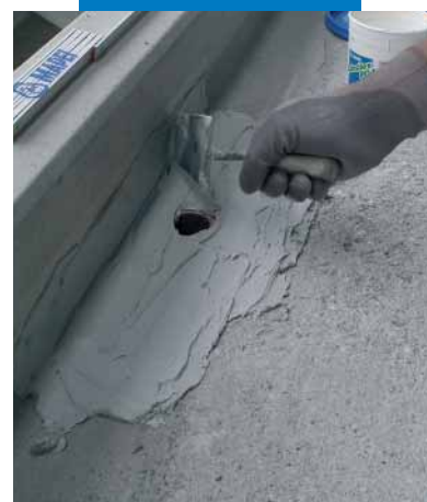
Final covering with Adesilex PG4
