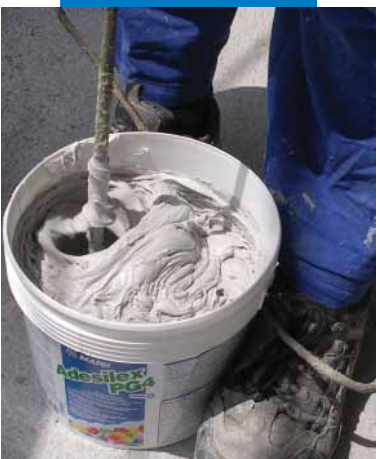
Preparing the mix
