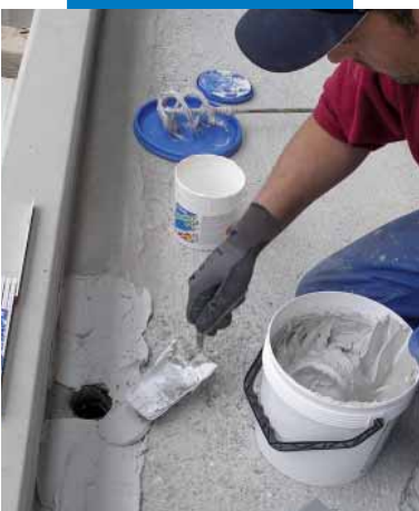
Applying Adesilex PG4 with a trowel
