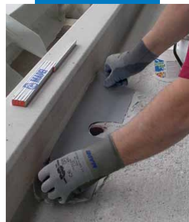
Laying flexible hyphalon brace
