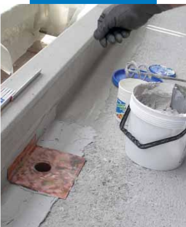
Laying a copper neck-flange and drain spout
